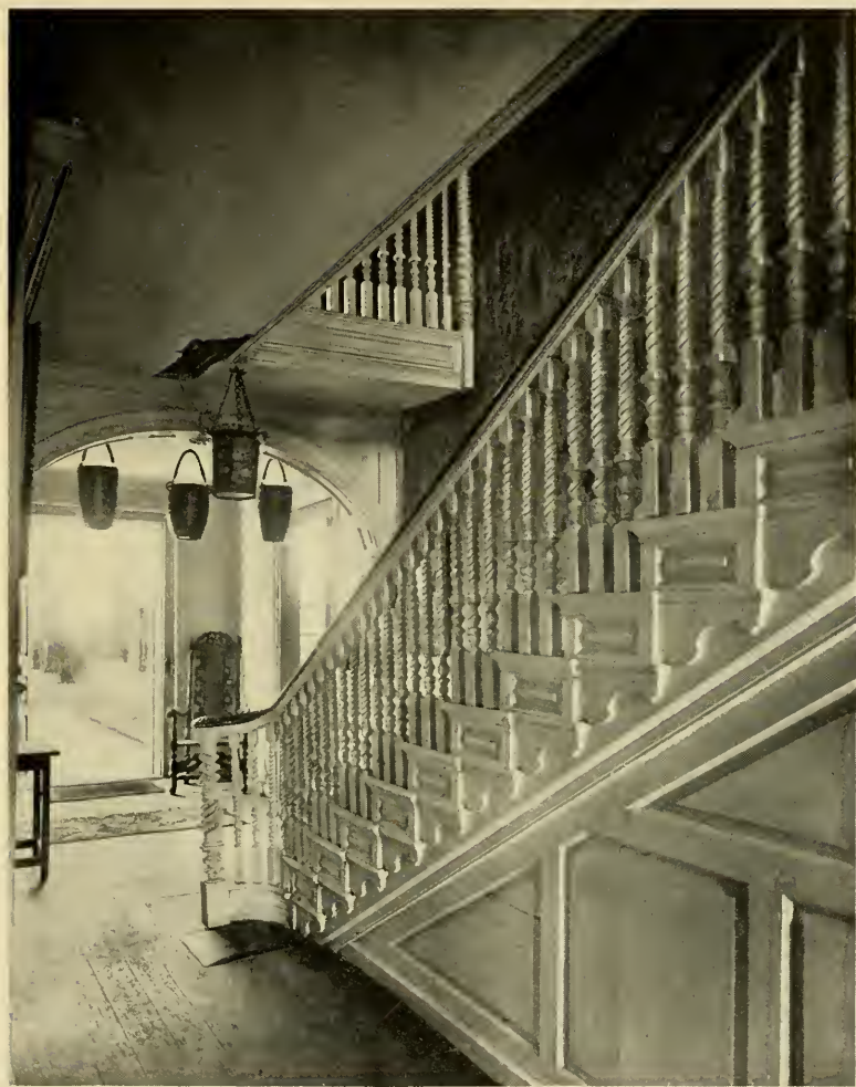
PLATE LXXX. — Hallway from the Rear, Royall House.
